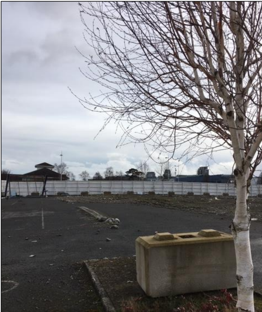
Figure 2: The Site which is dominated by hard standing (asphalt) with no vegetative establishment
